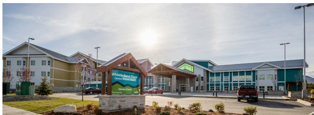
PHOTO CREDIT: PCL CONSTRUCTORS WESTCOAST INC.
